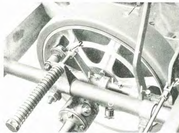
FRONT FLOOR BOARDS REMOVED (1).
