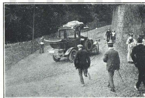
A Car on the Hill between Lynmouth and Lynton. Note the surface of the road, which is much worse higher up.
